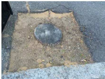
Removal of 8 tree stumps along West Street
