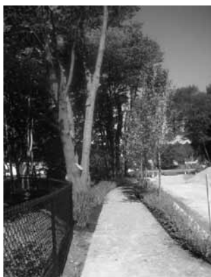
Newly installed pathway, planting and trees along Dix Way
