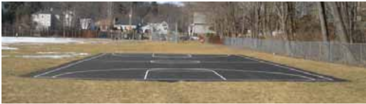
Newly repaired & re striped basketball court.
